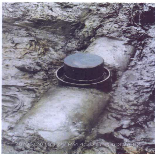
Fig B: picture taken after excavation.
